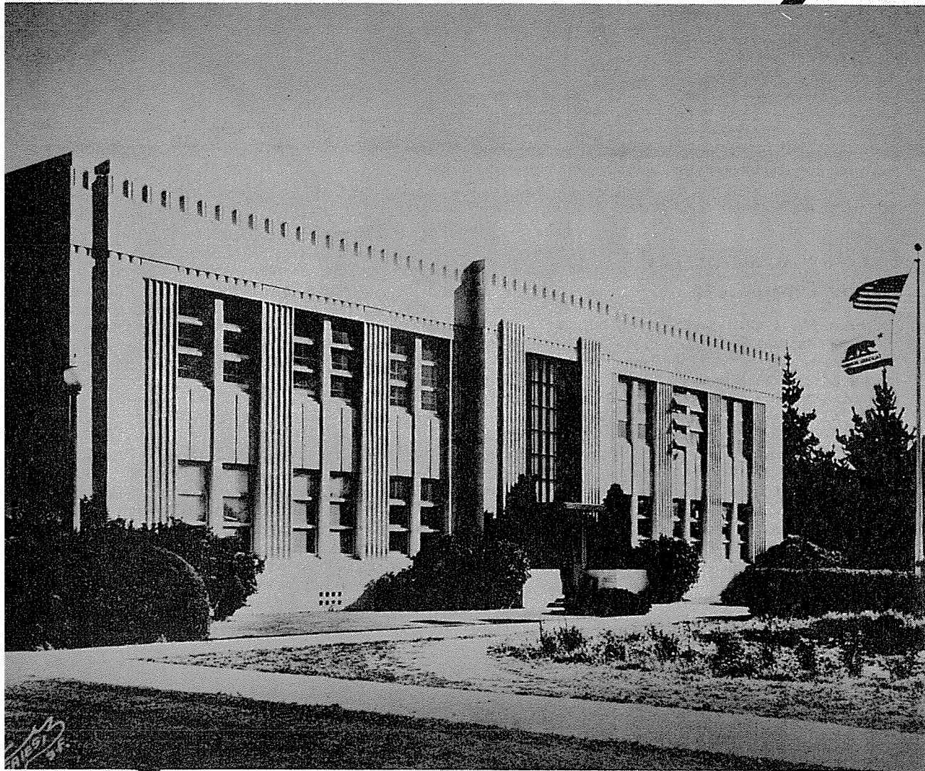
Science building is the first unit completed on the Delaware Campus in San Mateo.
